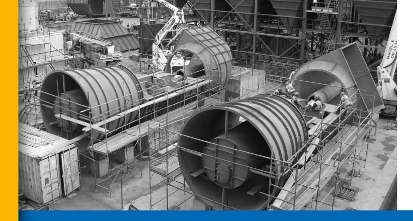
In the case of a conventional project design of a power plant, long-time proven, cost-effective, lowmaintenance and reliable Axial mixed flow fans, whose production and development has the longest tradition in ZVVZ, can be advantageously used.
