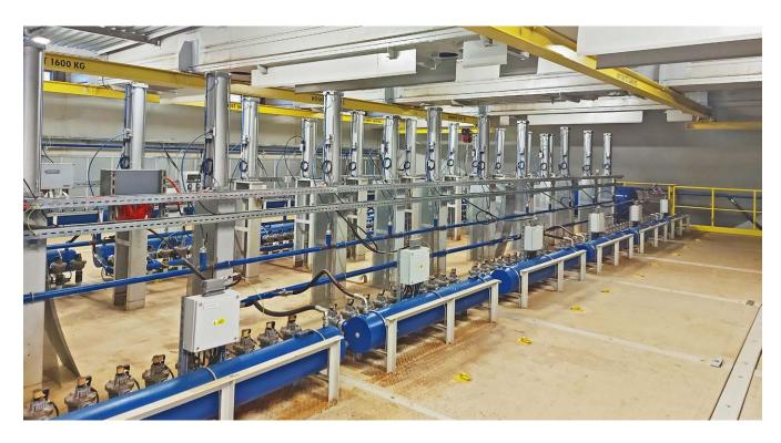
The specially designed regeneration system with venturi tube assures the high efficiency of regeneration with minimum consumption of compressed air. Compared to a system without an enclosed venturi tube, it generates four times the flow-rate and a pressure nearly three times greater on the internal surface of the filtration hose at the same pulse level, by drawing in additional clean gas.
