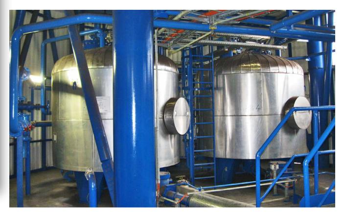
Chamber feeding devices are used in equipment for transporting larger amounts of loose materials over long distances. The throughput of equipment with chamber feeding devices may be (depending on the feeding device size) over a hundred tonnes per hour, with transport distances in the order of hundreds of metres.
